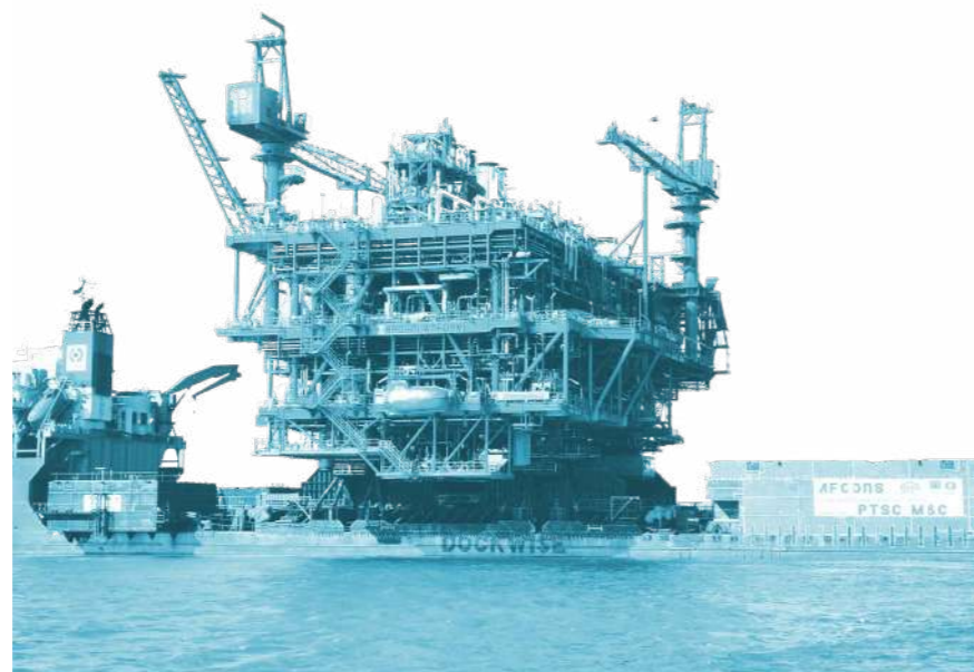
The HRD Offshore Platform Topside
