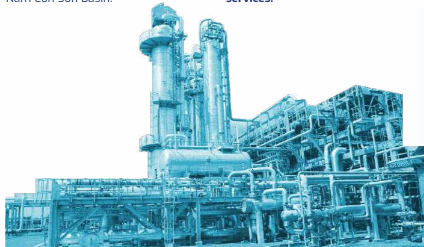
Dinh Co Gas Processing Plant Project (08/2001 - 02/2002)
